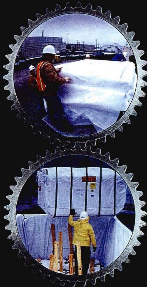
Our patented Lift Liner™ packaging may be the optimum answer to economic savings for some of your production operations and by-product waste operations. Photos show sludge and sediment removal operation that included; loading of materials into our versatile Lift Liner™ package, treatment, stabilization, hoisting into our private fleet of railcars and transport to final disposition.
